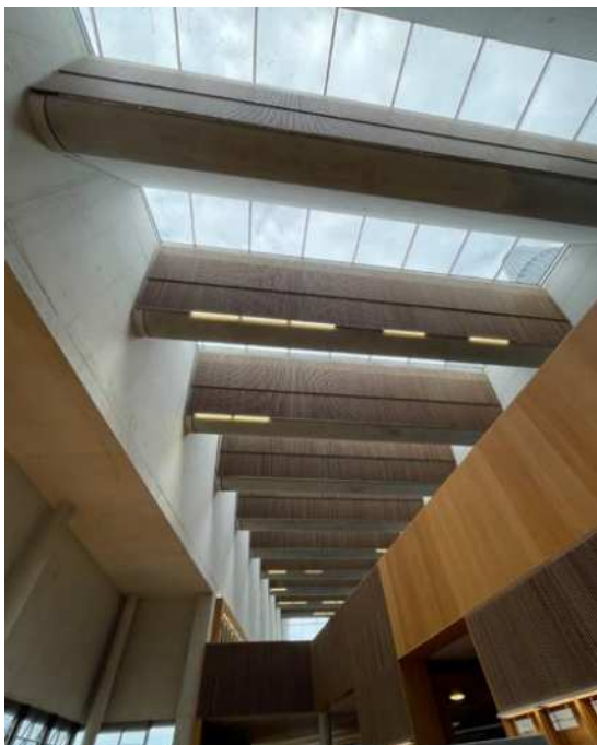
Figure 2: Precast concrete beams (Photo by BC)
