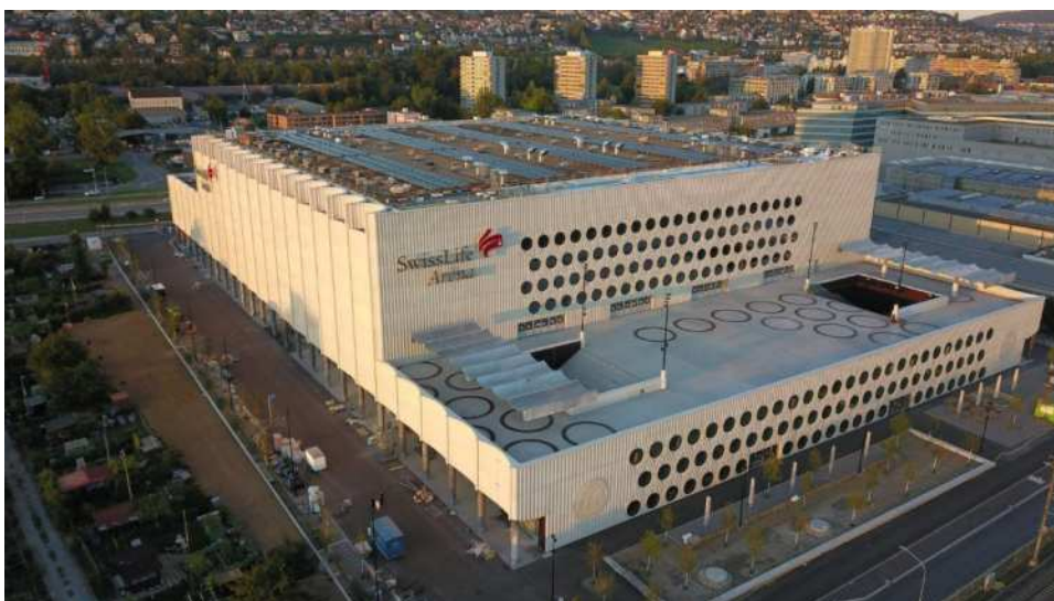
Figure 2. Swiss Life Arena with concrete cladding (Williams, 2022).
