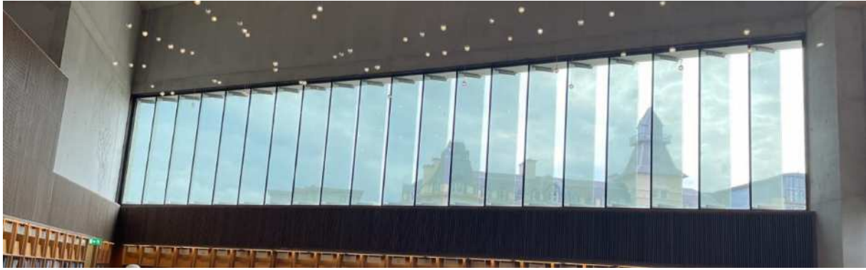
Figure 4: Window on internal face of wall (Photo by BC)
