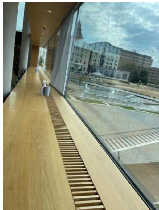
Figure 3: Window on external face of wall (Photo by BC)
