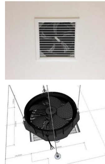
Detail of the integrated fan: view from below (left, upper) and from above (left, bottom). Shared office room with two integrated ceiling fans (right).
